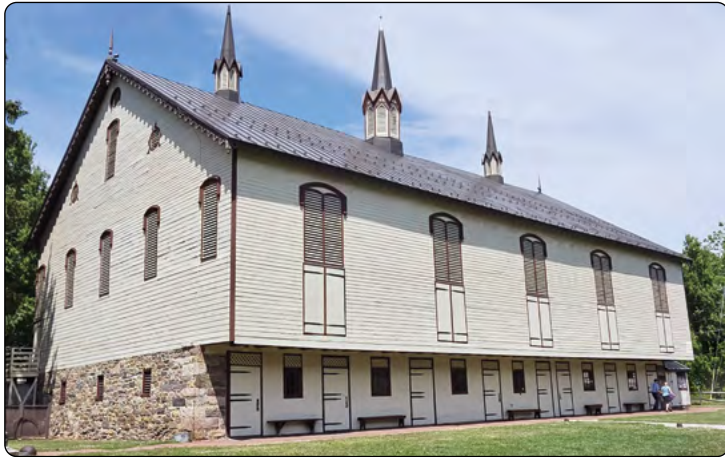
Centennial Barn at Fort Hunter in Harrisburg
