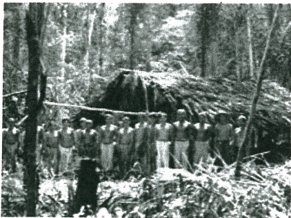
Workers clearing the rainforest before construction can begin
