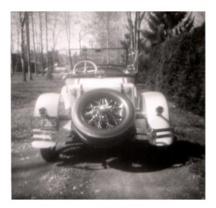
The Ford was a knockout, juice brakes, push button starter, Rajo heads, chrome covers on the wire wheel covers, running lights and dual spare tires with knock off hubs.
